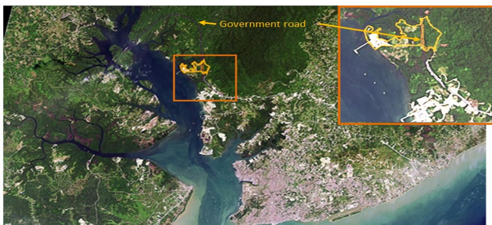
The PT WINA Industrial Site at Balikpapan and Government Road.
